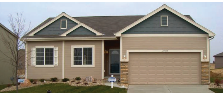
The Sheridan model displays one of the new exterior stone finishes, designed to create a warm and welcoming entry.
